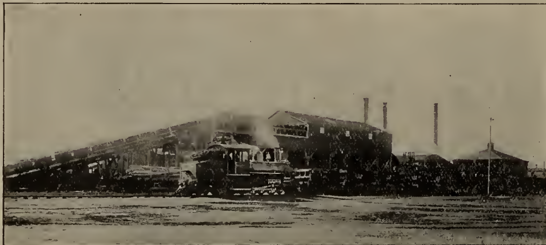
COLLIERIES AT WESTVILLE, NOVA SCOTIA.
